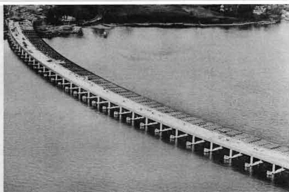
Concrete has been laid on one side of the causeway
