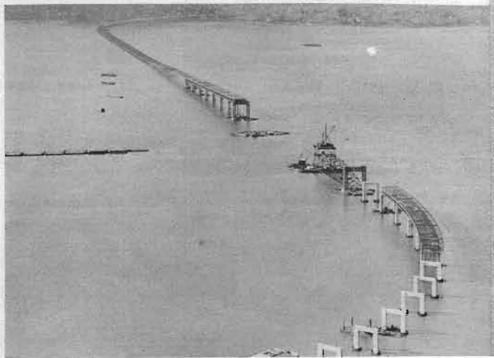
Gigantic trusses dwarf the tugboats that carefully jockey them into position Steelwork for the center span begins, with one of the pieces of falsework in place
