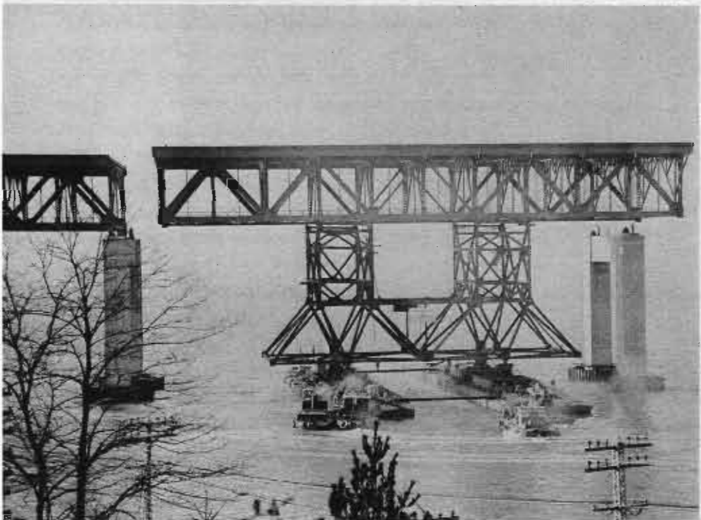
Bridge trusses being built at Haverstraw to be floated downstream, placed on piers Almost ready to be set down. Note men standing on the piers waiting for contact
