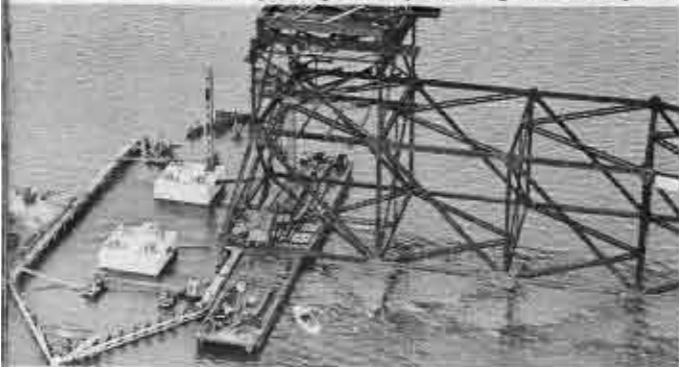
The first piece of steel goes into place
