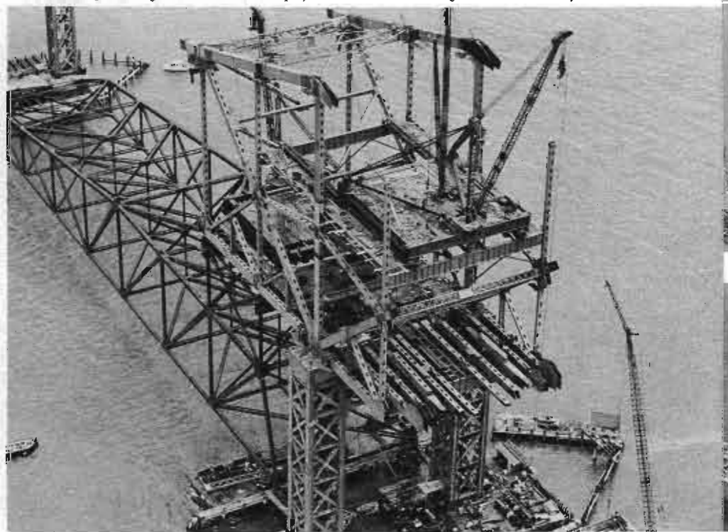
Falsework in place and the construction of the steel under-supports progresses Now the span begins to take shape, balanced securely on the steel falsework
