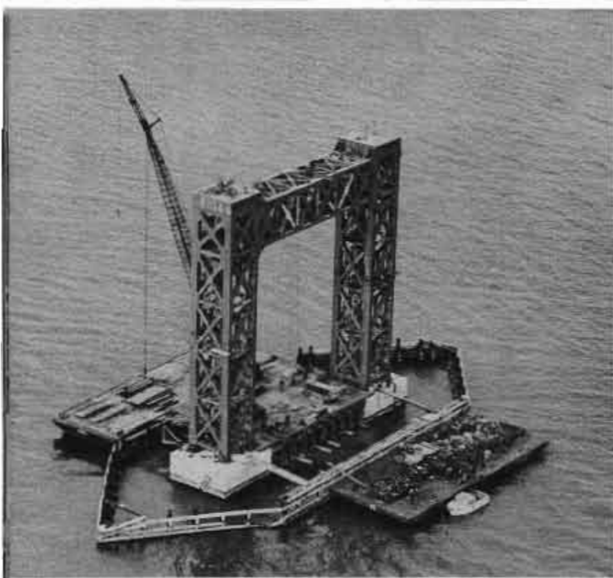
A steel pier to support the main span is almost completed
