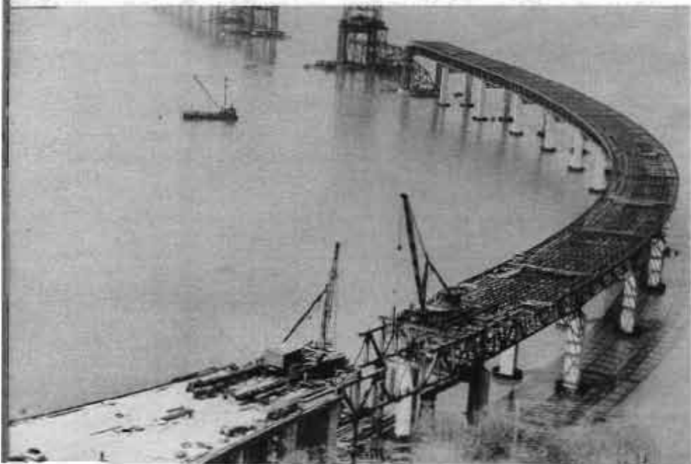
A steel pier to support the main span is almost completed
