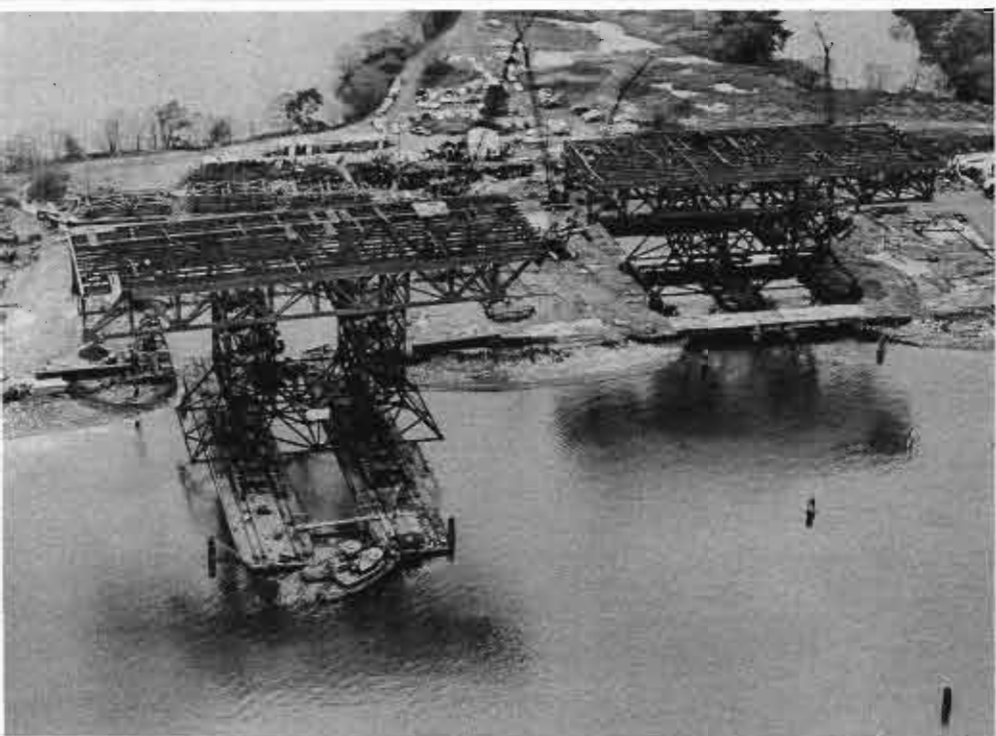
Bridge trusses being built at Haverstraw to be floated downstream, placed on piers Almost ready to be set down. Note men standing on the piers waiting for contact
