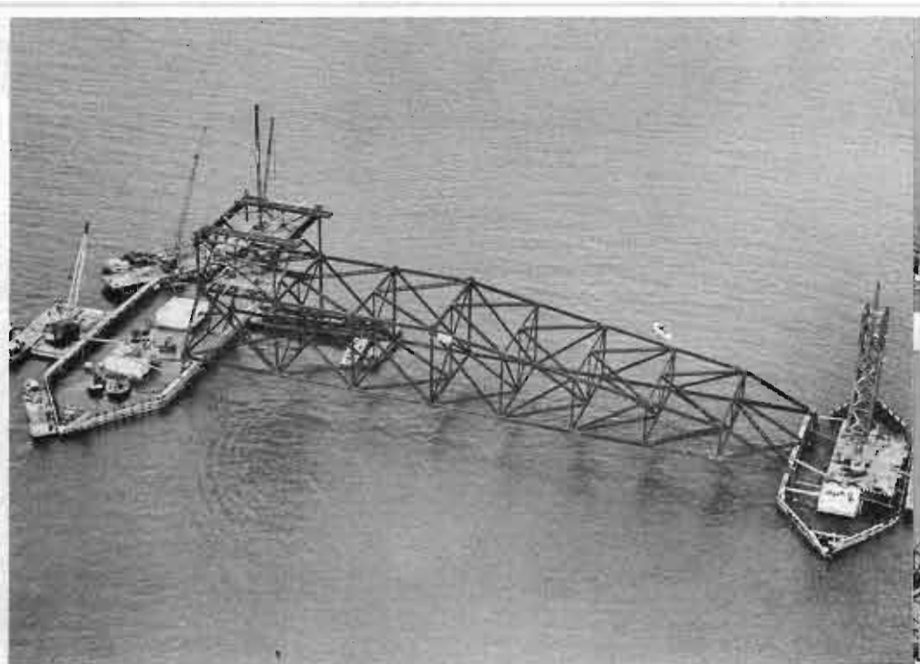
Falsework in place and the construction of the steel under-supports progresses Now the span begins to take shape, balanced securely on the steel falsework
