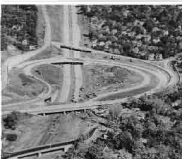
Approach from west shore under construction
