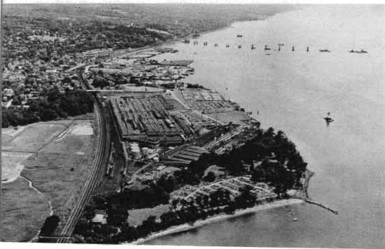
The bridge begins to take form. Chevrolet and Fisher Body plants are seen in foreground
